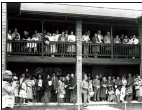
1992: Staff apartments built.
